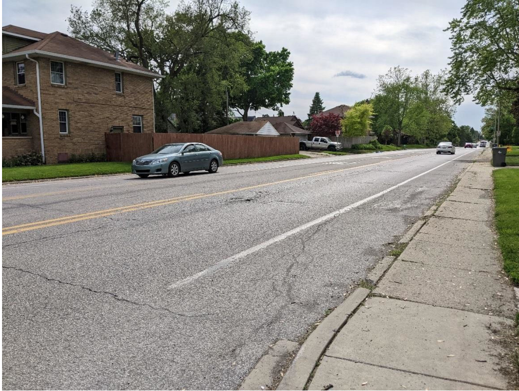
Figure 51. Photo of the northwest corner of 10 th and Audubon, looking west
