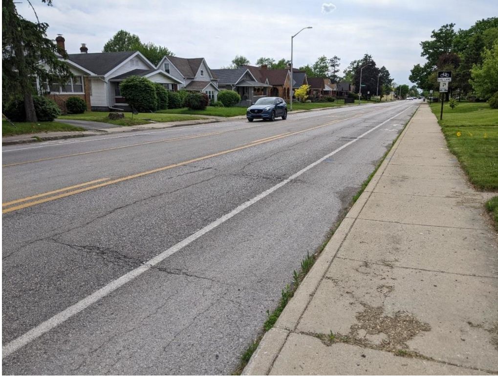
Figure 27. Photo of the southeast corner of 10 th and Hawthorne, looking west
