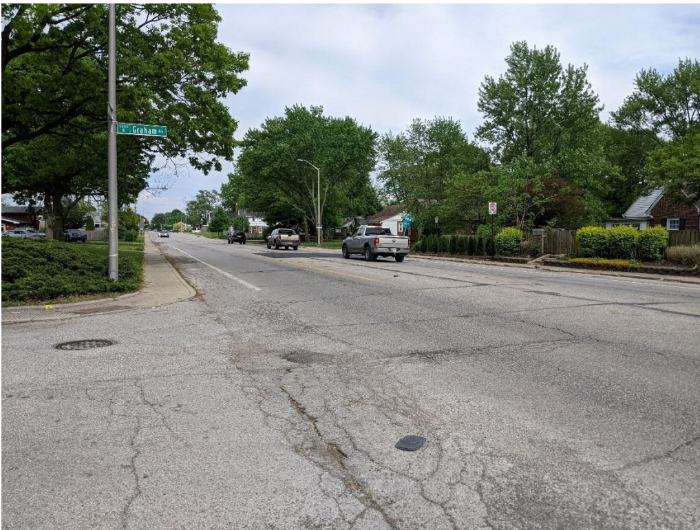
Figure 54. Photo of the northwest corner of 10 th and Graham, looking east
