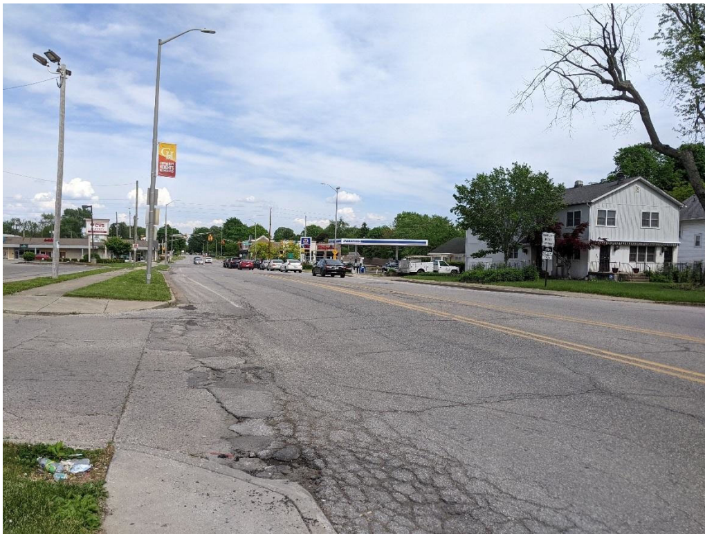
Figure 62. Photo of the northwest corner of 10 th and Campbell, looking east
