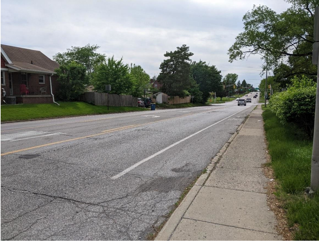
Figure 43. Photo of the northwest corner of 10 th and Layman, looking west
