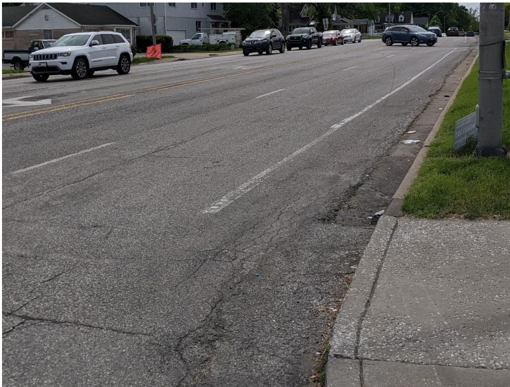
Figure 66. Photo of the northwest corner of 10 th and Arlington, looking east
