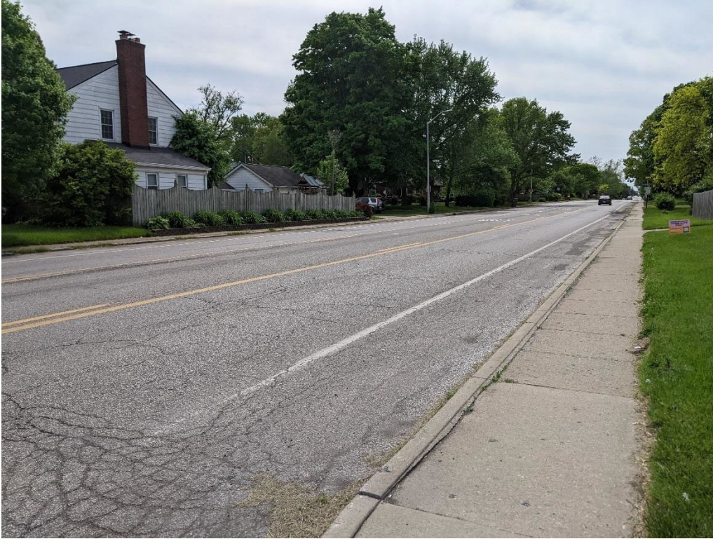
Figure 59. Photo of the northwest corner of 10 th and Bolton, looking west
