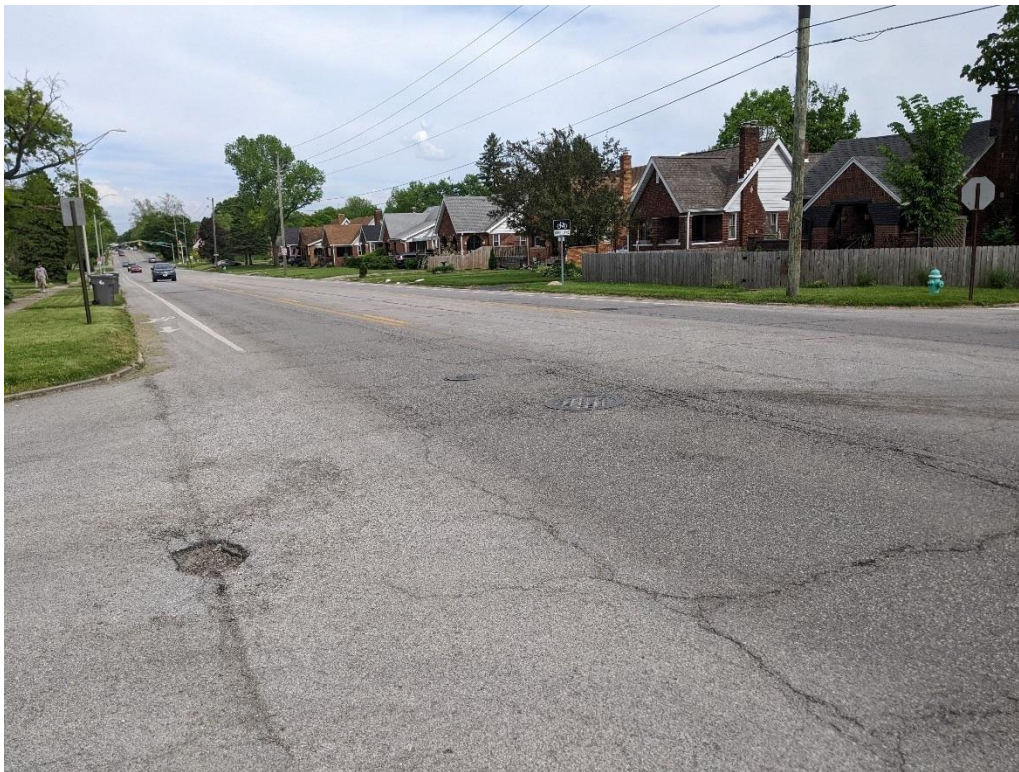
Figure 32. Photo of the northwest corner of 10 th and Irvington, looking east
