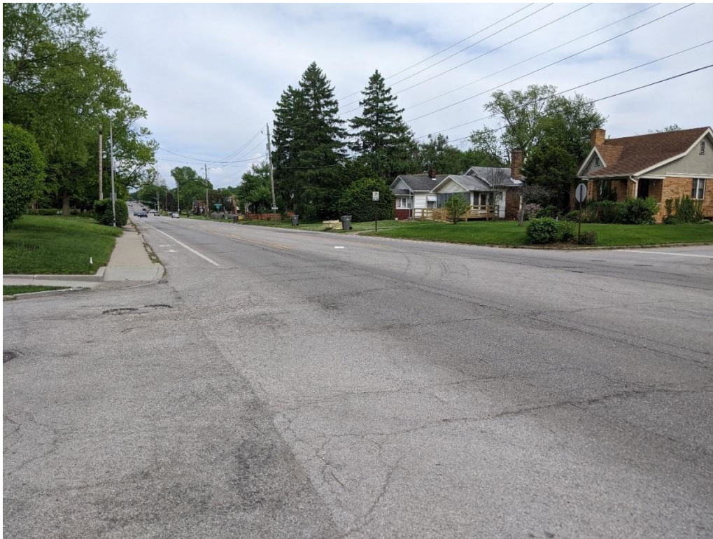
Figure 28. Photo of the northwest corner of 10 th and Downey, looking east
