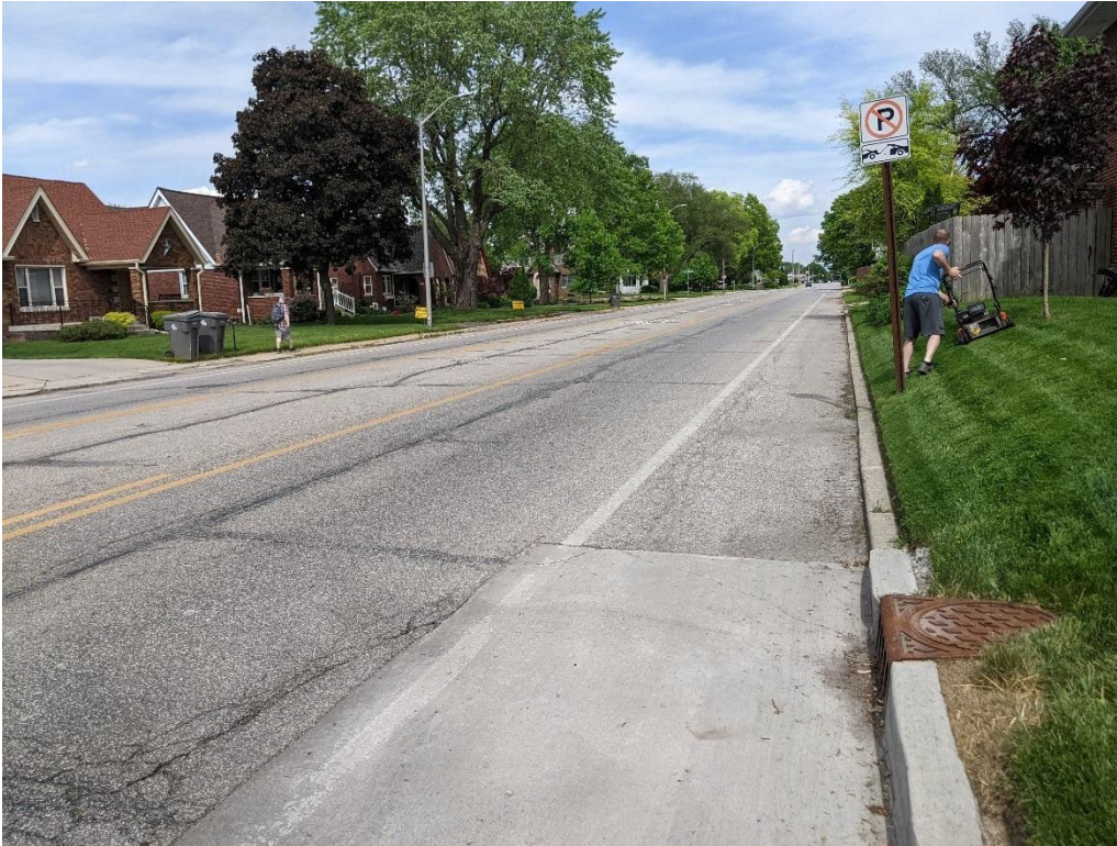
Figure 48. Photo of the southeast corner of 10 th and Lesley, looking east
