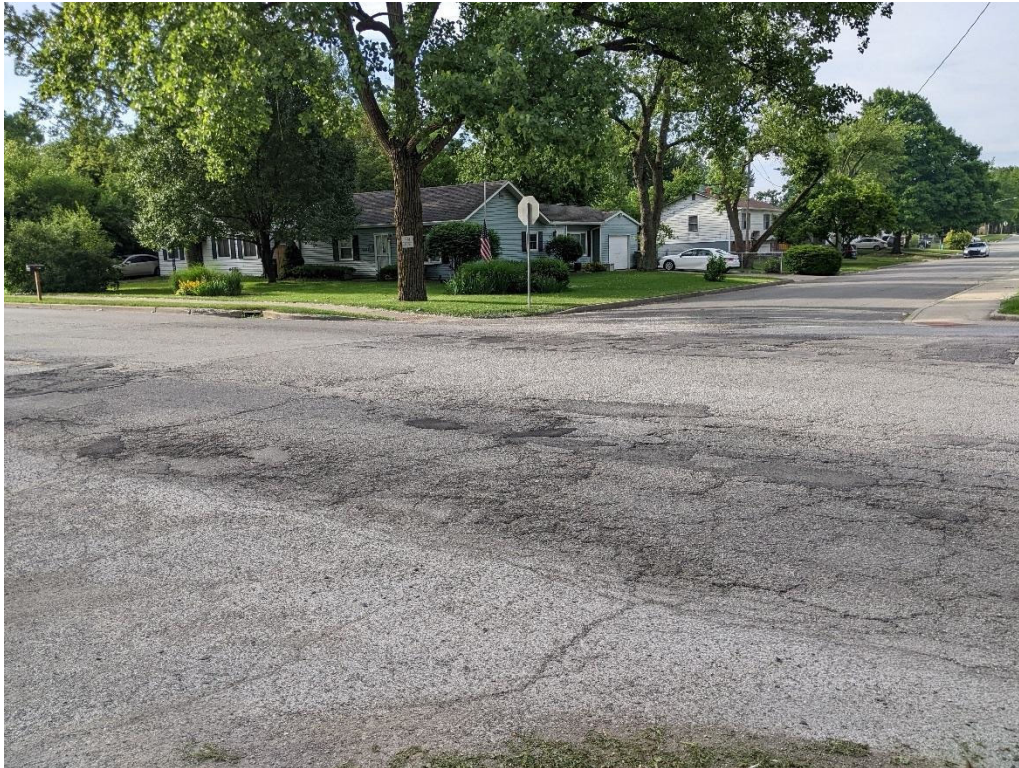
Figure 3. Photo of the northwest corner of 16 th and Bolton, looking east
