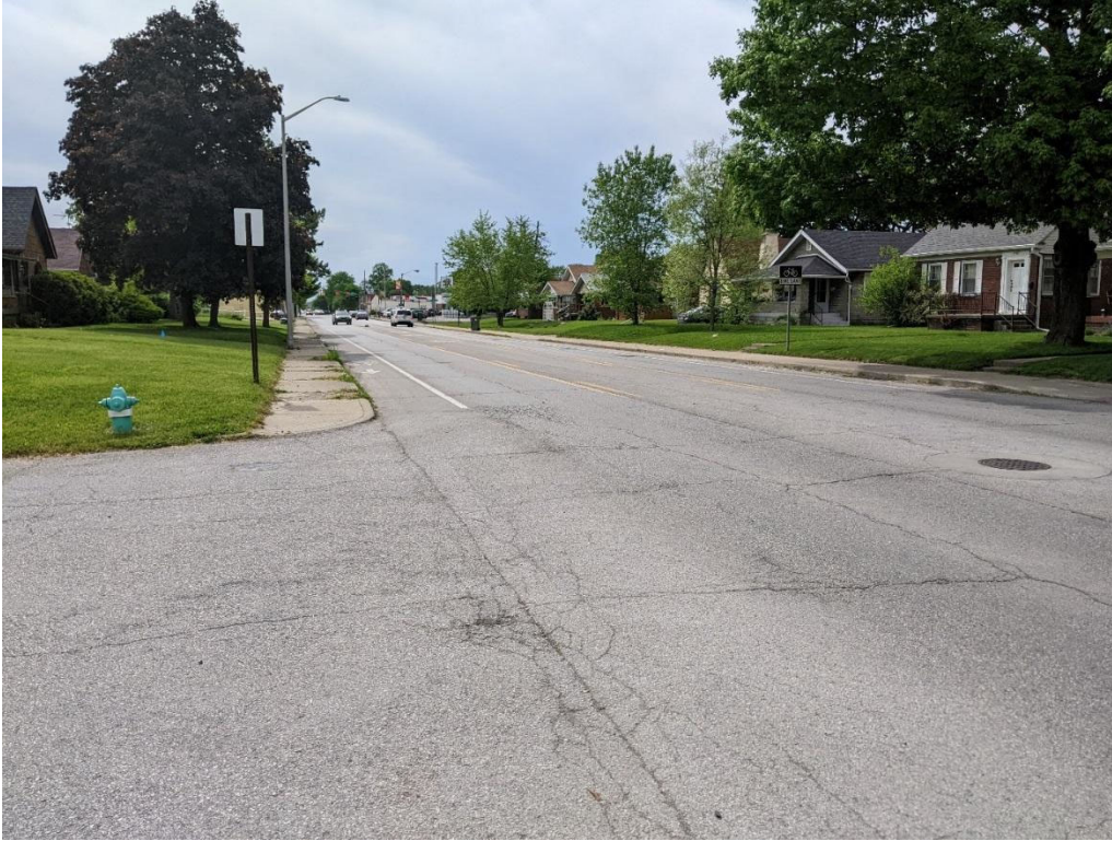
Figure 23. Photo of the southeast corner of 10 th and Butler, looking west
