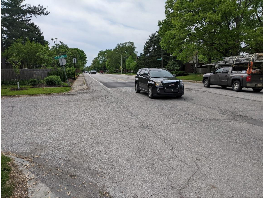
Figure 57. Photo of the southeast corner of 10 th and Graham, looking west
