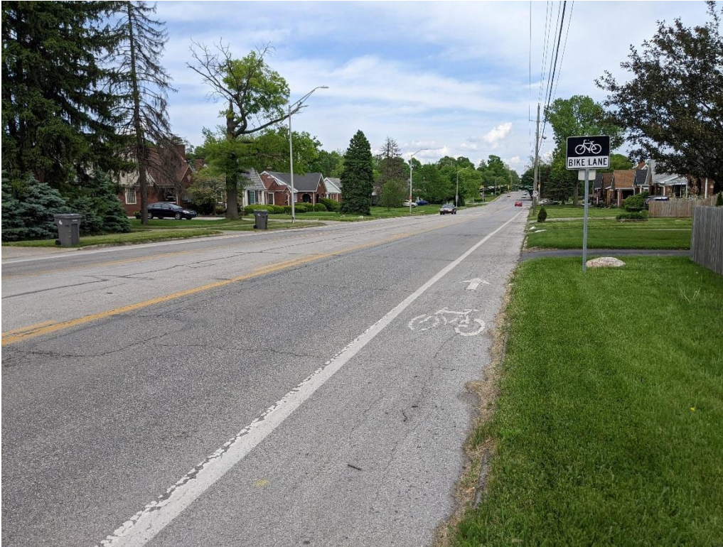
Figure 34. Photo of the southeast corner of 10 th and Irvington, looking east
