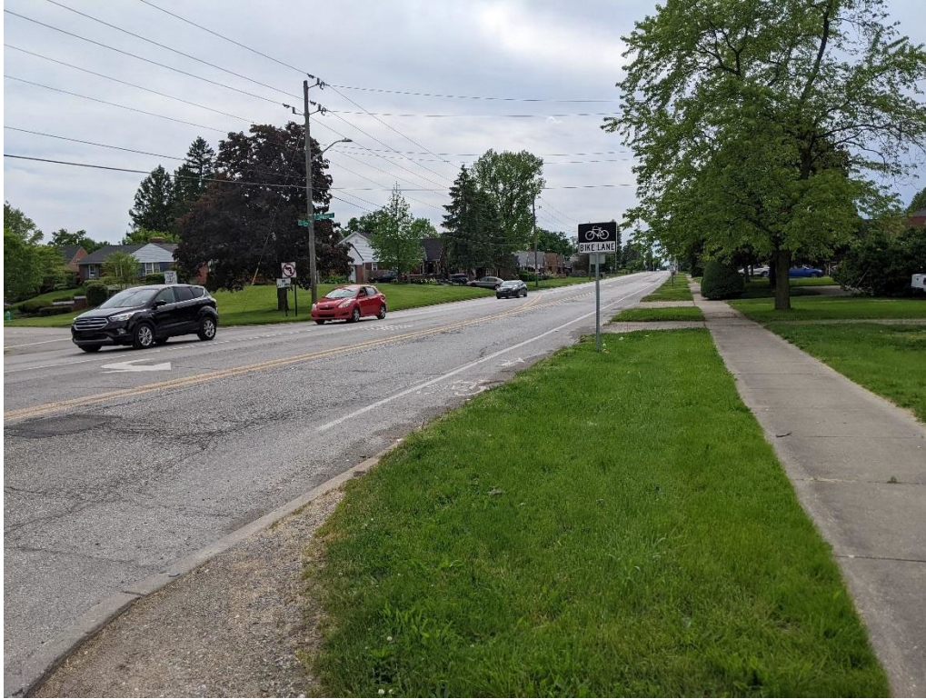
Figure 39. Photo of the northwest corner of 10 th and Ritter, looking west
